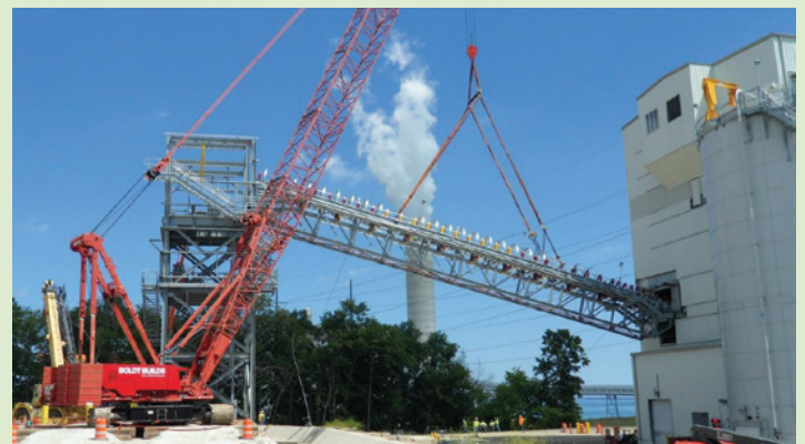
A crane lifts a conveyor truss from a transfer tower to a drive tower at Elm Road Generating Station.
