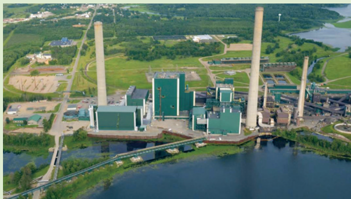
Boswell Energy Center Unit 4
