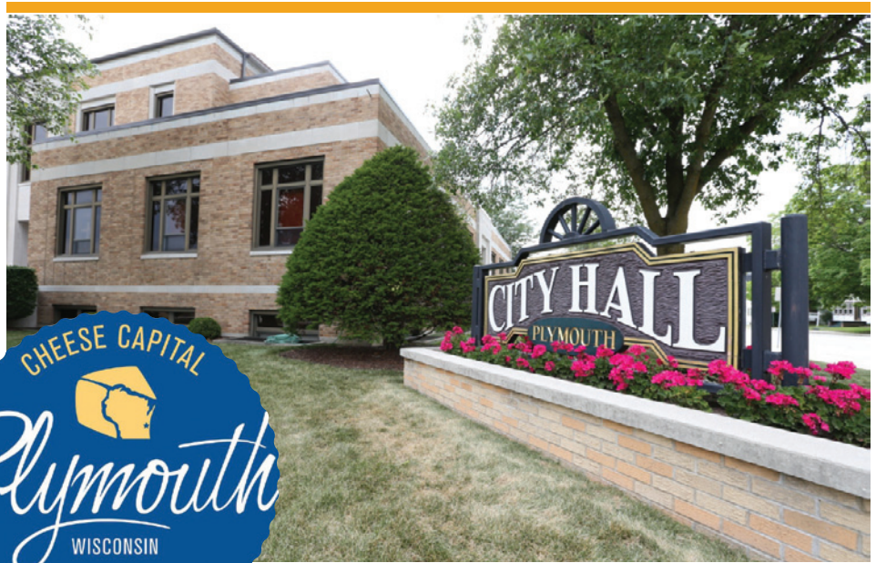
Plymouth City Hall is installing rooftop solar panels to offset part of the building's energy usage.
